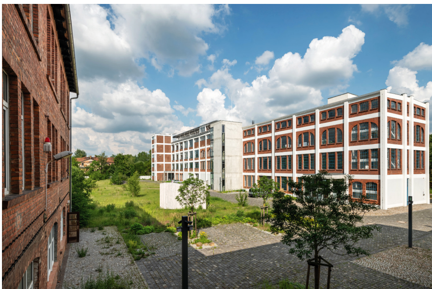
Built by Bauhaus architect Egon Eiermann, today's industrial monument is home to the Thuringian Center for Telemedicine. Photo: © Thomas Müller
